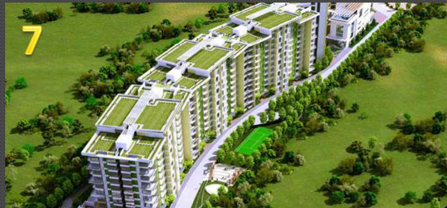
Project: Nitesh Columbus Square Location: Bellary Road Area: 0.56 Mn Sqft
